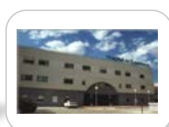
HOSPITAL DE SALAMANCA (General d Inversions Tormes, S.A)
